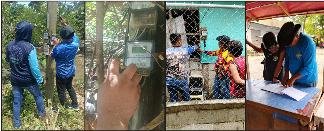
Testing and replacement of defective kWh meters.
